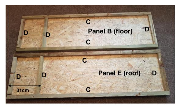
3) Position another baton (D) 31cm from one end and screw through panel (B) into baton using 2 screws.
